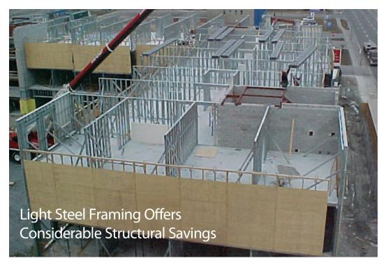
Kingsway Arms Retirement Home is a 6-storey, 160-unit, 9,890 m<sup>2</sup> (106,456 ft<sup>2</sup>) facility located at the corner of Eglinton and McCowan in the Scarborough area of eastern Toronto. It was constructed in 14 months using panelized light steel framing (LSF), with a stone veneer and stucco exterior. Developer-builder The Rockport Group attributes significant savings to the LSF system's versatility.
