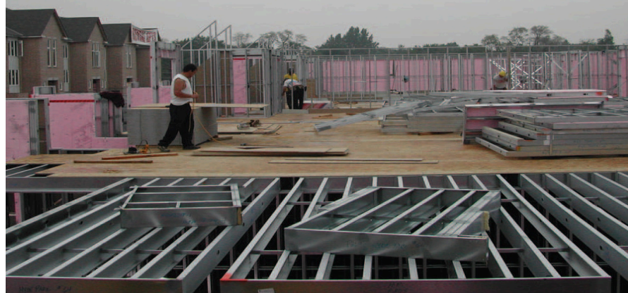
Hyde Park Condominiums (Zentil): Genesis TM steel panels and roof trusses made from light steel framing contribute significantly to meeting several of the prime building considerations - quality, lightweight and speed of erection.
