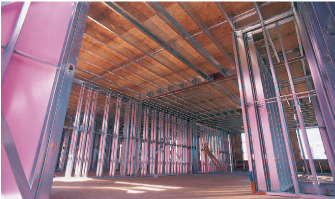
King West Village (Urbancorp): Extensive use of light steel framing, both structural LSF sections and non-loadbearing, was a feature of this four-storey project.
