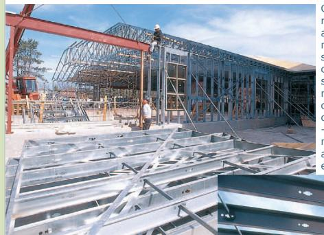
Genesis<sup>™</sup> steel roof trusses and wall panels made from light steel framing contributed significantly to meeting several of the prime considerations - light weight, noncombustibility and speed of erection.
